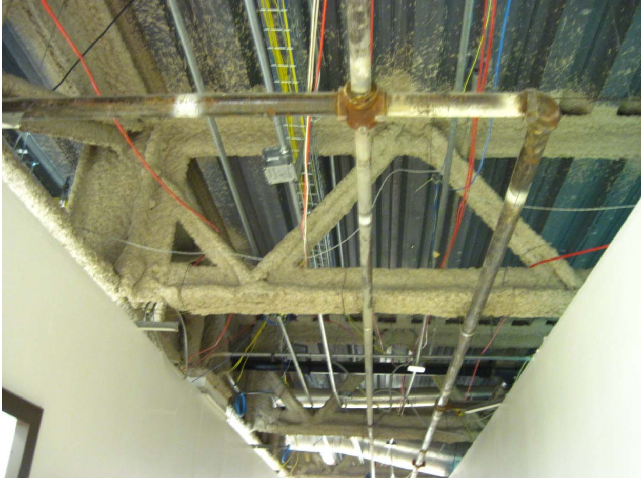
Figure 9: An example of a truss that will be reinforced
