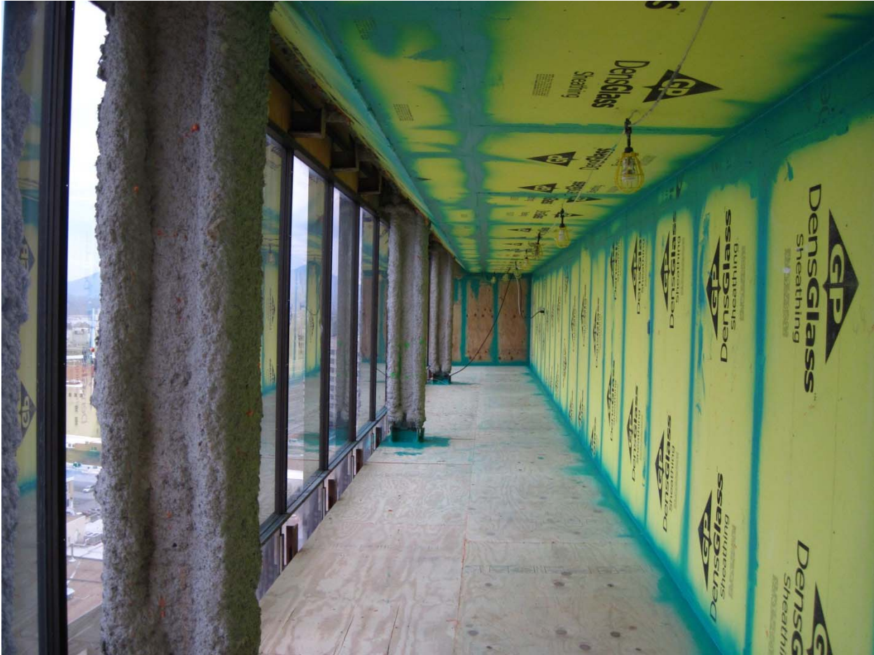
Figure 6: Temporary weather wall
