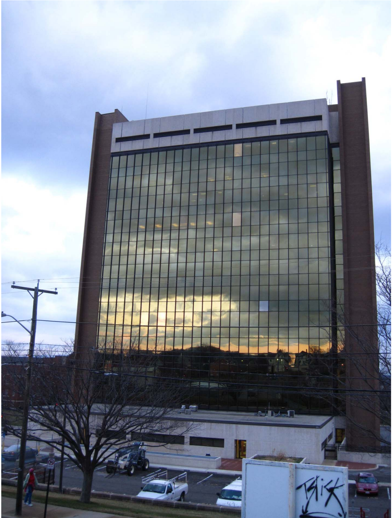
Figure 35: Photo of South-facing façade of the Government Office Center
