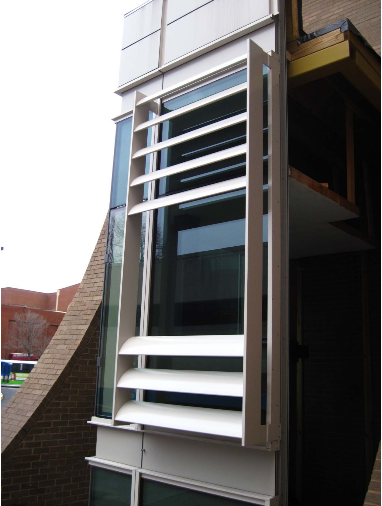
Figure 33: Photo of the curtain wall mockup at the GOC
