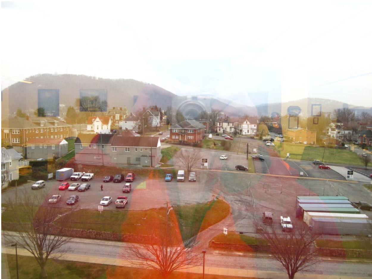
Figure 34: Photo from the South-facing existing curtain wall
